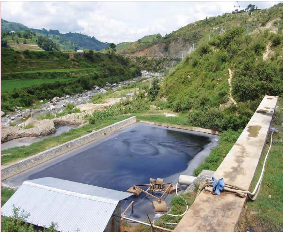
Leachate treatment systems form one of the key elements for upgrading landfill practices, Ghorahi, Nepal
