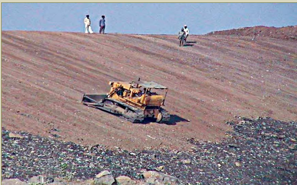
Fencing and levelling of the dumpsite for upgrading
