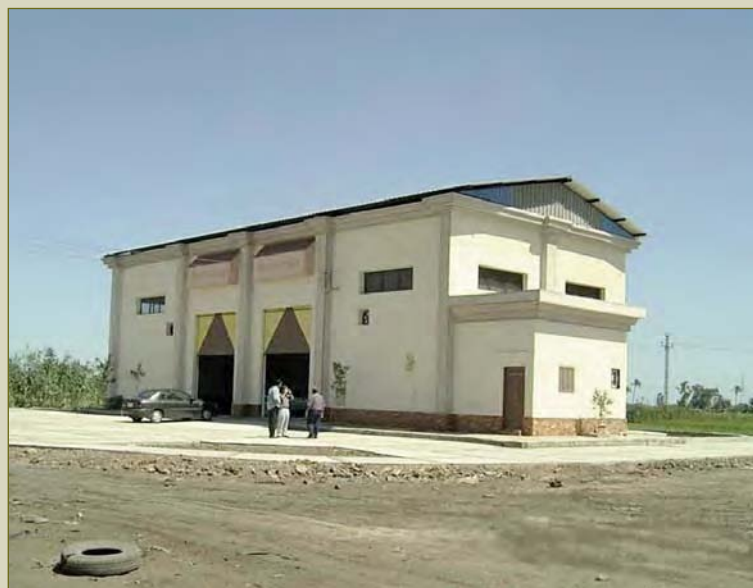
Transfer station at Faraskour, Egypt. The design is suitable for up to 150 tonnes/day capacity
