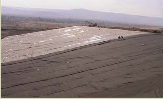
Laying HDPE liner
