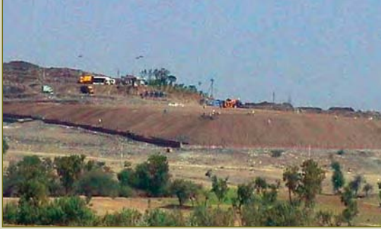
Covering of the old dumpsite while dumping is continu- ing in adjacent area
